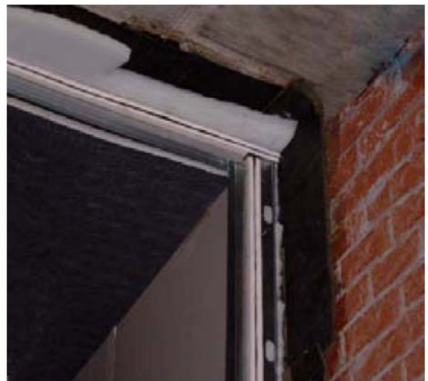
Partition wall and ceiling insulation with LA
