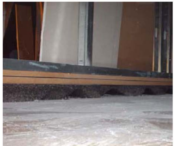
Floating floor with LA-10.
