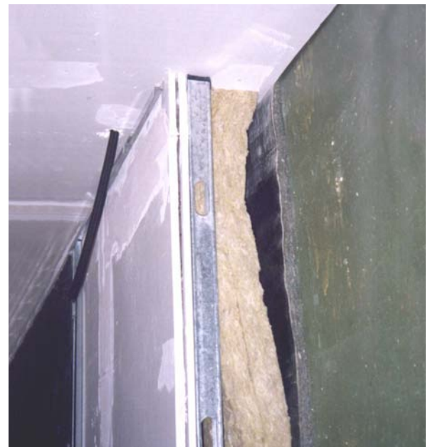
Partition wall insulation with PKB-2.
