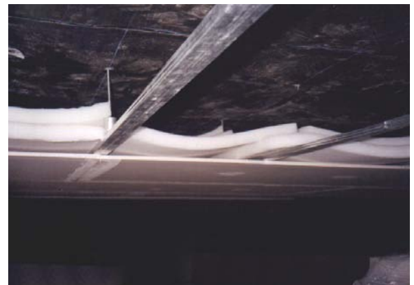
Ceiling insulation with PKB-2
